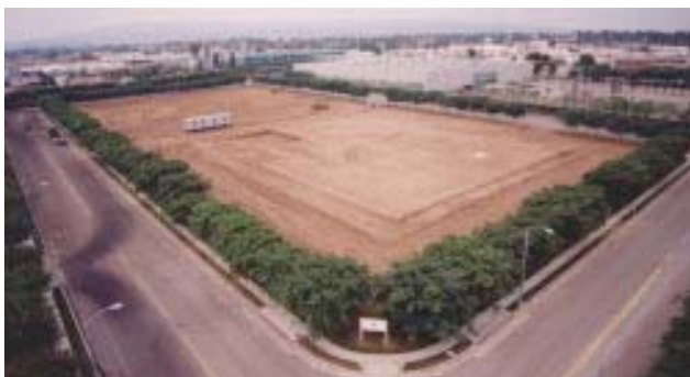
New Sakura Finetek U.S.A. headquarters site leveled and ready for foundations.
