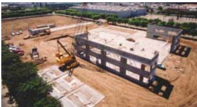
Walls and superstructure going up on schedule.
